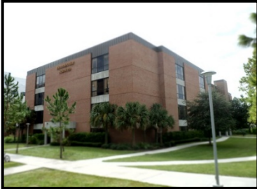
Biomedical Sciences Building, Main Campus
