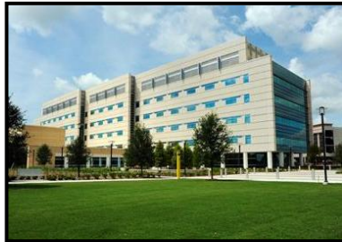
Burnett Biomedical Sciences Building, Health Sciences Campus
