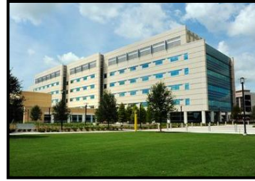
Burnett Biomedical Sciences Building, Health Sciences Campus
