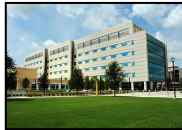
Burnett Biomedical Sciences Building, Health Sciences Campus
