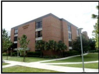
Biomedical Sciences Building, Main Campus
