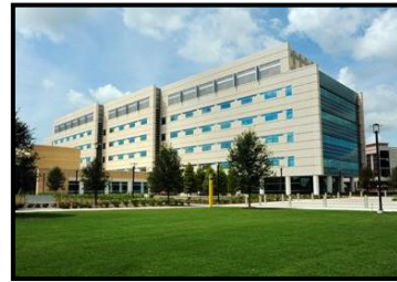
Burnett Biomedical Sciences Building, Health Sciences Campus
